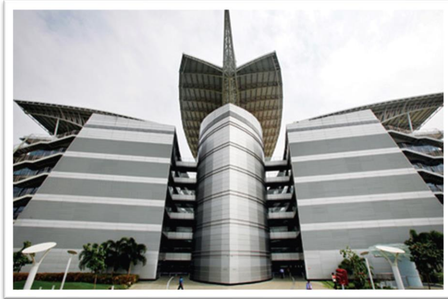
Tata Consultancy Services building in SIPCOT, Siruseri.
