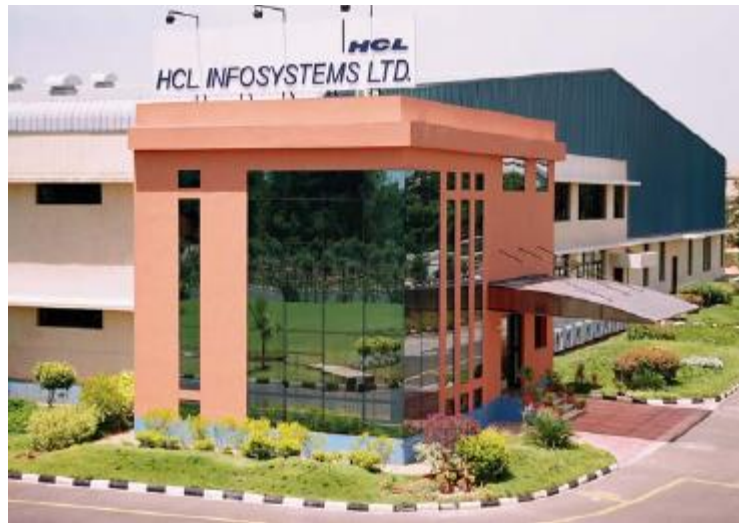
HCL Production Facility
