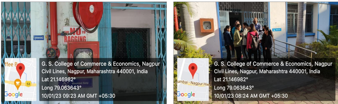
On-site review with the team for fire and life safety systems
