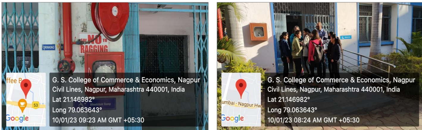
On-site review with the team for fire and life safety systems
